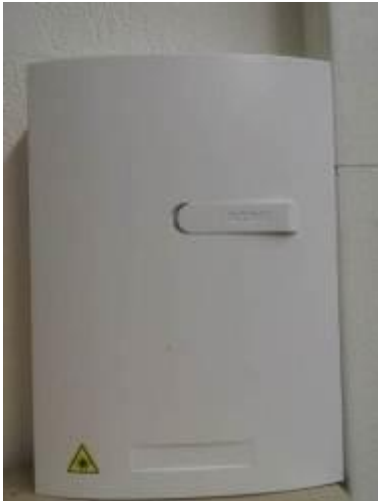
Figure 10 : PBO ACOME mono fibre
